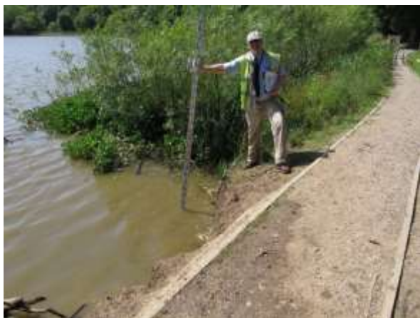
Erosion damage to the dam of Great Pond on Epsom Common LNR caused by dogs. autumn 2012 repairs cost £18500
